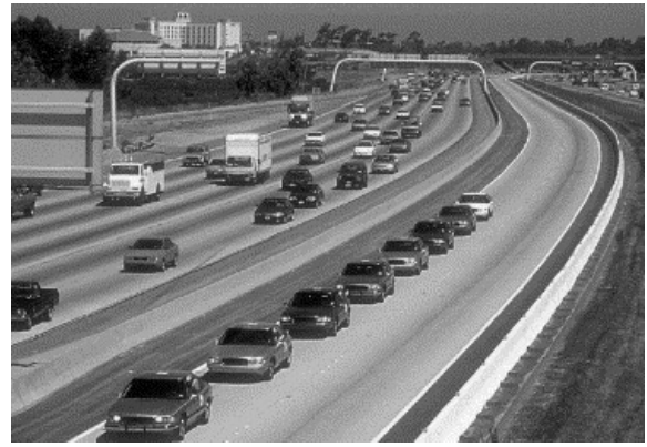
(b) PATH: Testing an eight car automated platoon on an Automated Highway System(1997)
